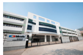
TELEHOUSE HONG KONG CCC
