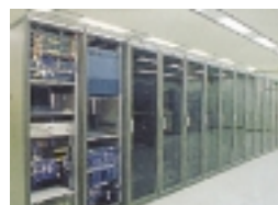
Interior of colocation room (KDDI Building, Shinjuku)
