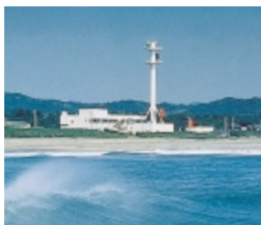
Chikura Cable Landing Station
