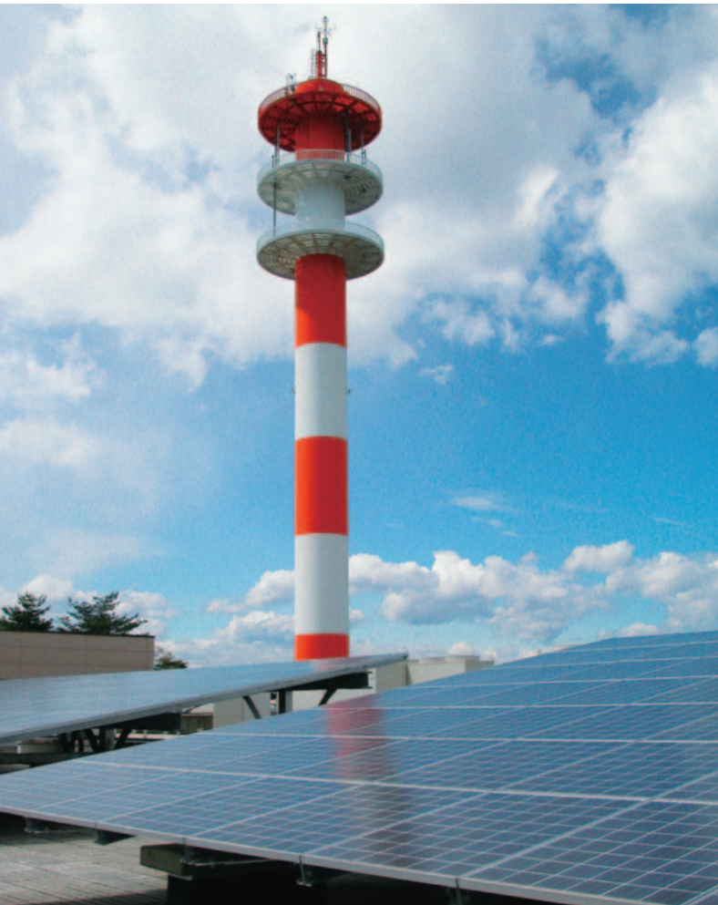
Solar panels at the Oyama Network Center. These support clean energy in KDDI's telecommunications services.
