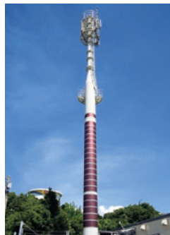
Amorphous solar cells base station
