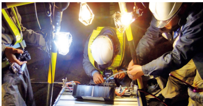
Communication cable recovery work on backbone routes
