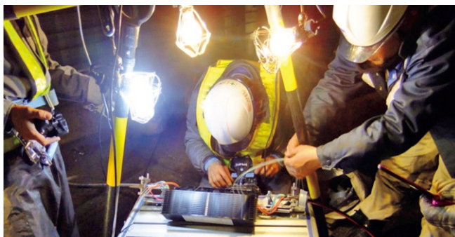
Communication cable recovery work on backbone routes
