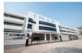
TELEHOUSE HONG KONG CCC
