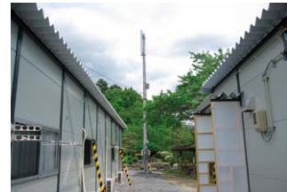
New au mobile phone base station installed near temporary housing
