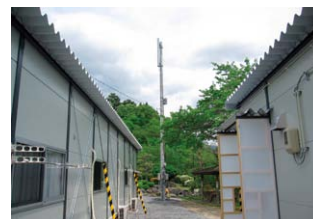
New au mobile phone base station installed near temporary housing
