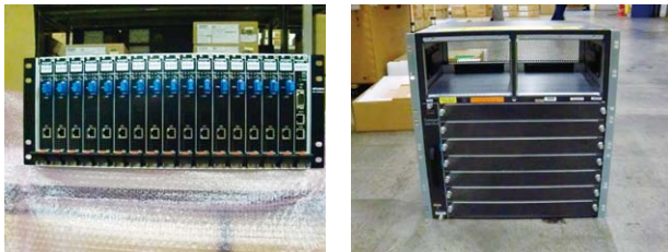
Subscriber communications network base station terminating equipment (left) and data transfer equipment in temporary storage at a resource management center Storage racks (right)
