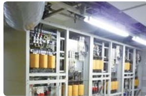
Former 800MHz frequency base station power source
