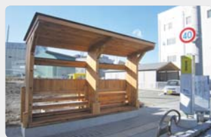
Bus shelter made from thinned materials
