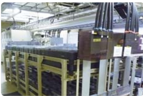
Former 800MHz frequency base station battery (storage battery)
