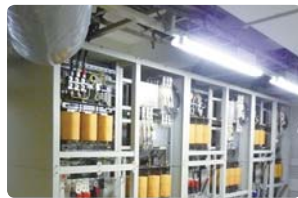
Former 800MHz frequency base station power source
