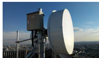
Radio Transmission Path Relay Station
