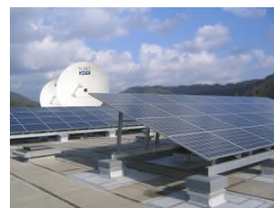
Large scale communications station using natural energy
