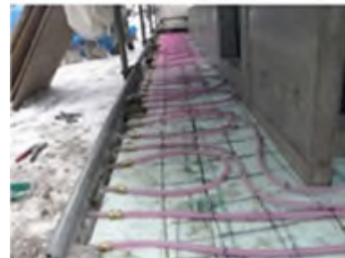
Road heating facilities
