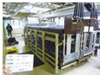
Former 800MHz frequency base station storage battery
