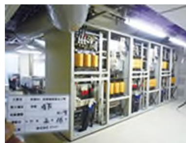
Former 800MHz frequency base station power source
