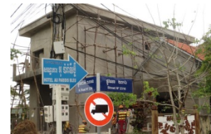
Relay station under construction (Cambodia)
