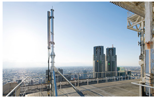
One of the wide-zone base station antennas on the roof of KDDI Office Building Shinjuku
