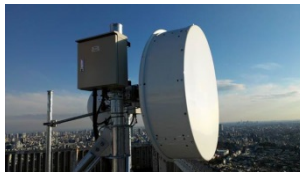
Radio Transmission Path Relay Station
