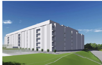
Simulated image of TELEHOUSE TOKYO Tama 3 building
