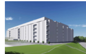
Exterior view of TELEHOUSE TOKYO Tama 3
