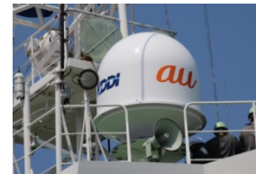
The experimental mobile phone base station is installed on the bridge of the patrol vessel Satsuma.
