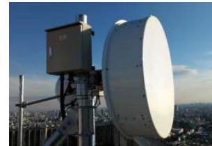
Radio Transmission Path Relay Station
