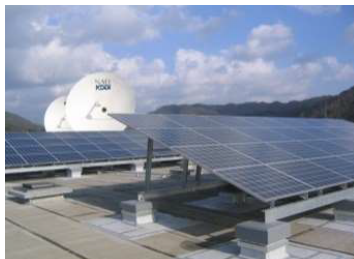
Large scale communications station using natural energy
