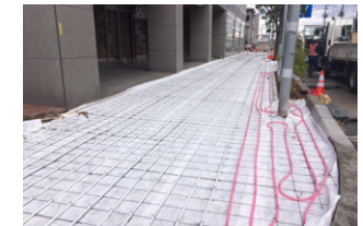
Road heating facilities
