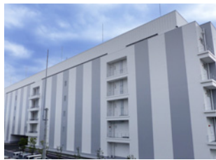
TELEHOUSE TOKYO Tama 3 exterior
