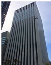
TELEHOUSE OSAKA 2 exterior
