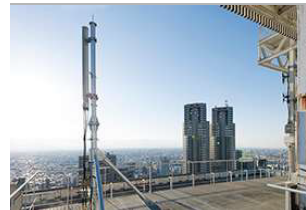
One of the wide-zone base station antennas on the roof of KDDI Office Building Shinjuku
