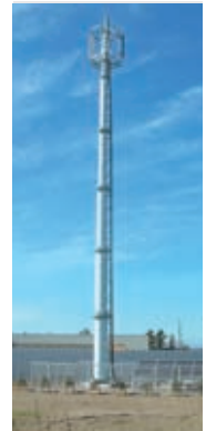
au mobile phone base station employing “tribrid” power control technology
