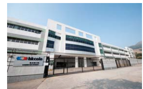
TELEHOUSE HONG KONG CCC
