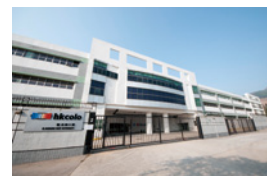
TELEHOUSE HONG KONG CCC
