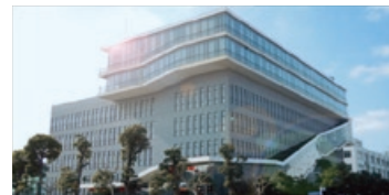
TELEHOUSE上海 JinQiao (金橋)
