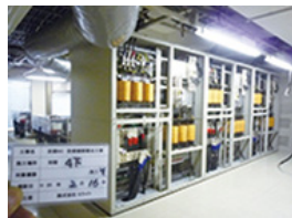
Former 800MHz frequency base station power source
