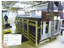
Former 800MHz frequency base station storage battery
