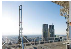
One of the wide-zone base station antennas on the roof of KDDI Office Building Shinjuku
