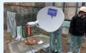
Satellite femtocell: Ishinomaki, Miyagi Pref.
