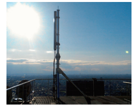
One of the wide-zone base station antennas on the roof of the KDDI Building in Shinjuku
