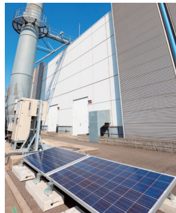
Tribrid base station
