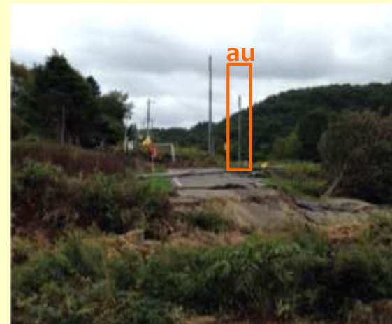
[Hokkaido Eastern Iburi earthquake] Base station facilities were isolated
