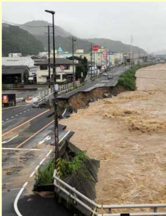
[Torrential rain in July 2018] Optical cable disconnection
