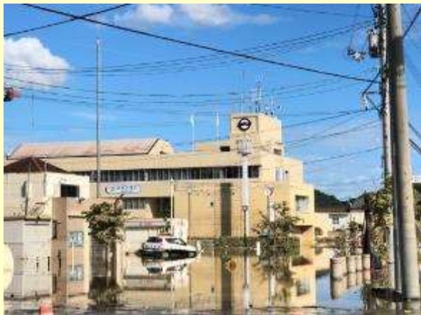
[Torrential rain in July 2018] Network Center was flooded
